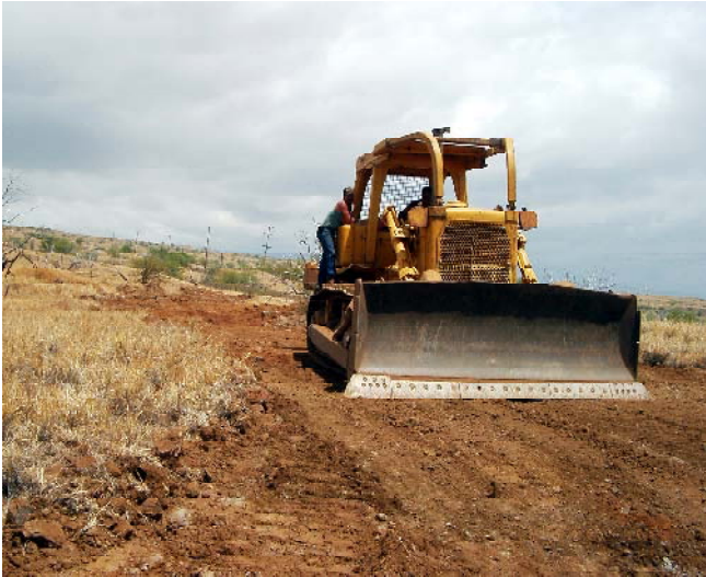
Photo: Fire Break Construction
